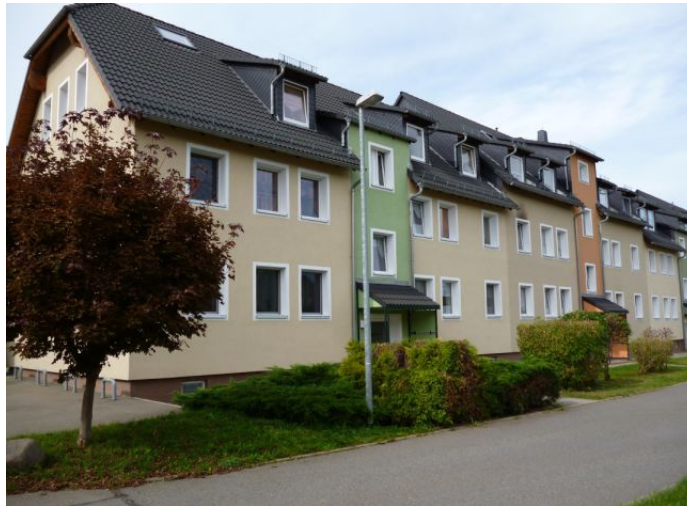
Picture 2: Block of flats after selective redevelopment and modernisation, designated for rented flats.
